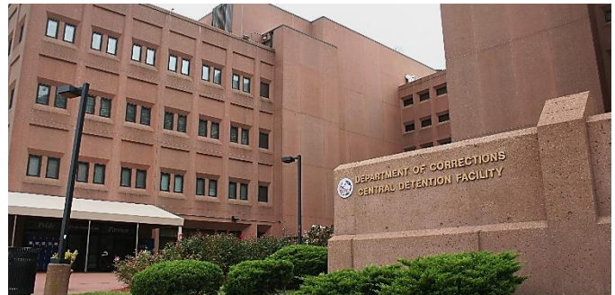
Central Detention Facility (CDF)
