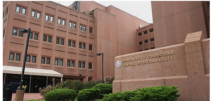
Central Detention Facility (CDF)
