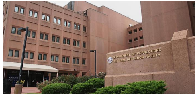
Central Detention Facility (CDF)
