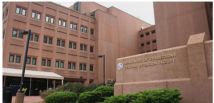
Central Detention Facility (CDF)
